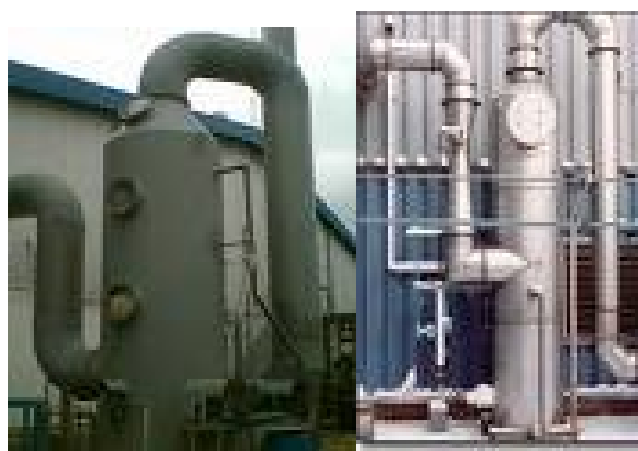
Figura 09 – Torre ou coluna absorvedora (Scrubber)
